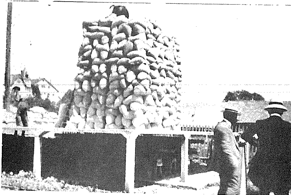
MAILLART NINE-BAY TEST FLOOR 1908
