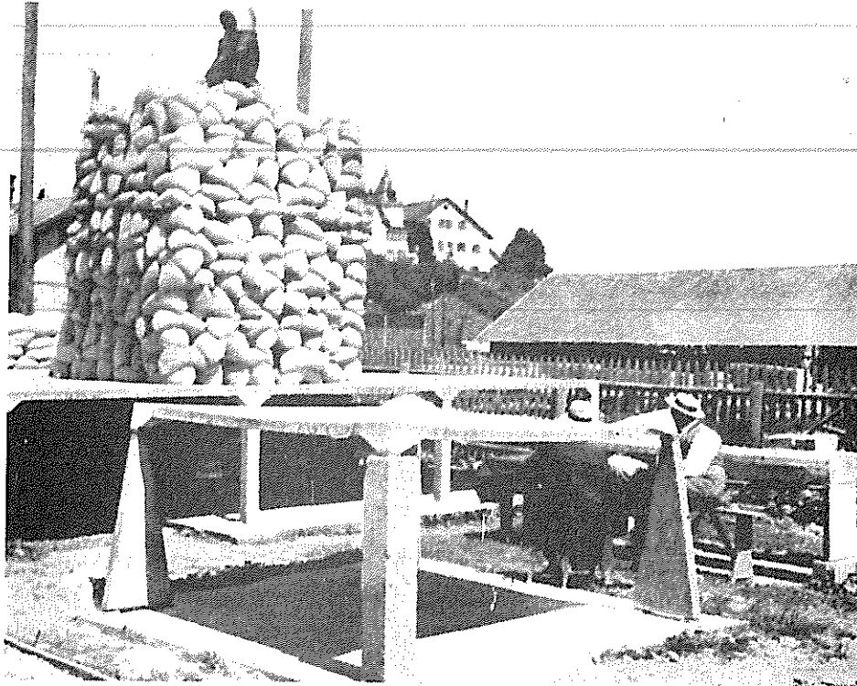
MAILLART TEST SLABS 1908
