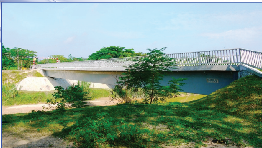
World's longest span reactive powder box girder bridge
