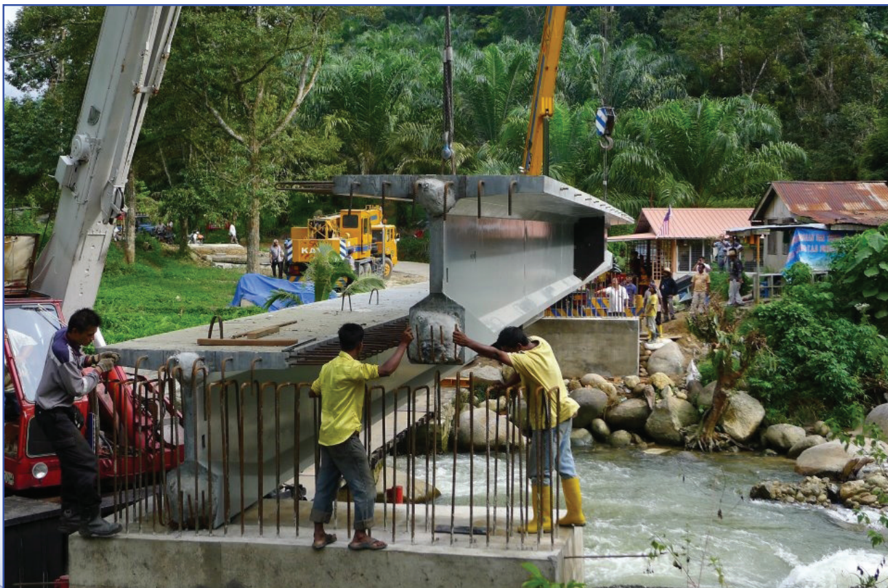
Pictures supplied by Dr. Voo. Ultra High-Performance, Reactive Powder, Concrete finds its way to the villages of Malaysia.
